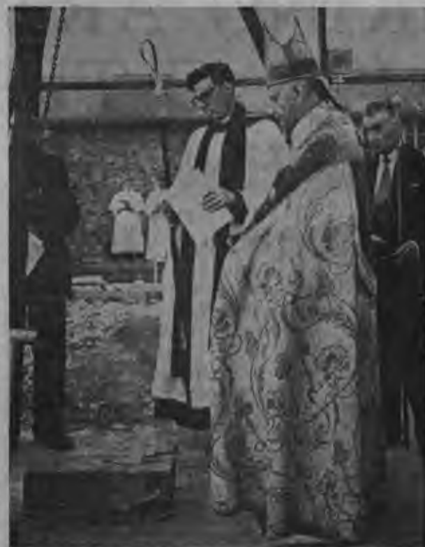
The Bishop of Lincoln, Rt. Rev. Kenneth Riches, lays the foundation stone of the Church of St. John the Baptist, on Ermine Estate, Lincoln. The stone, which is taken from Lincoln Cathedral, is unusually placed, being in the centre of the church.
